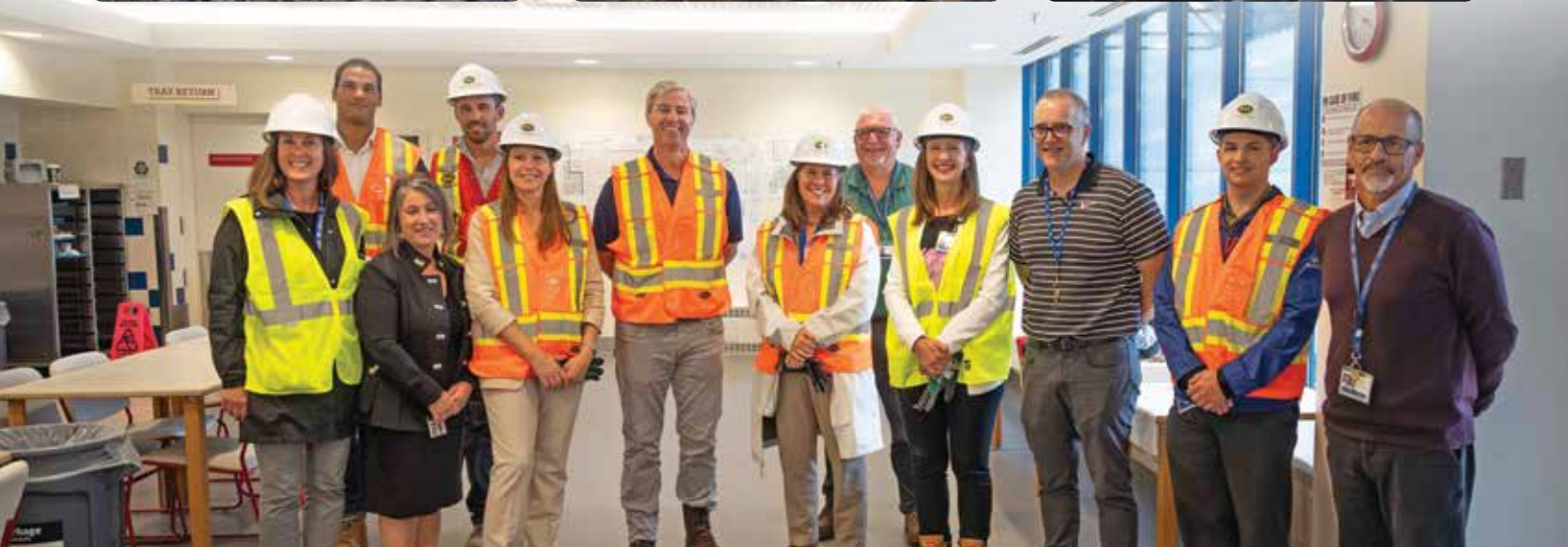
Premier Tim Houston tours SSRH redevelopment construction with Nova Scotia Health and Health Services Foundation leaders.
